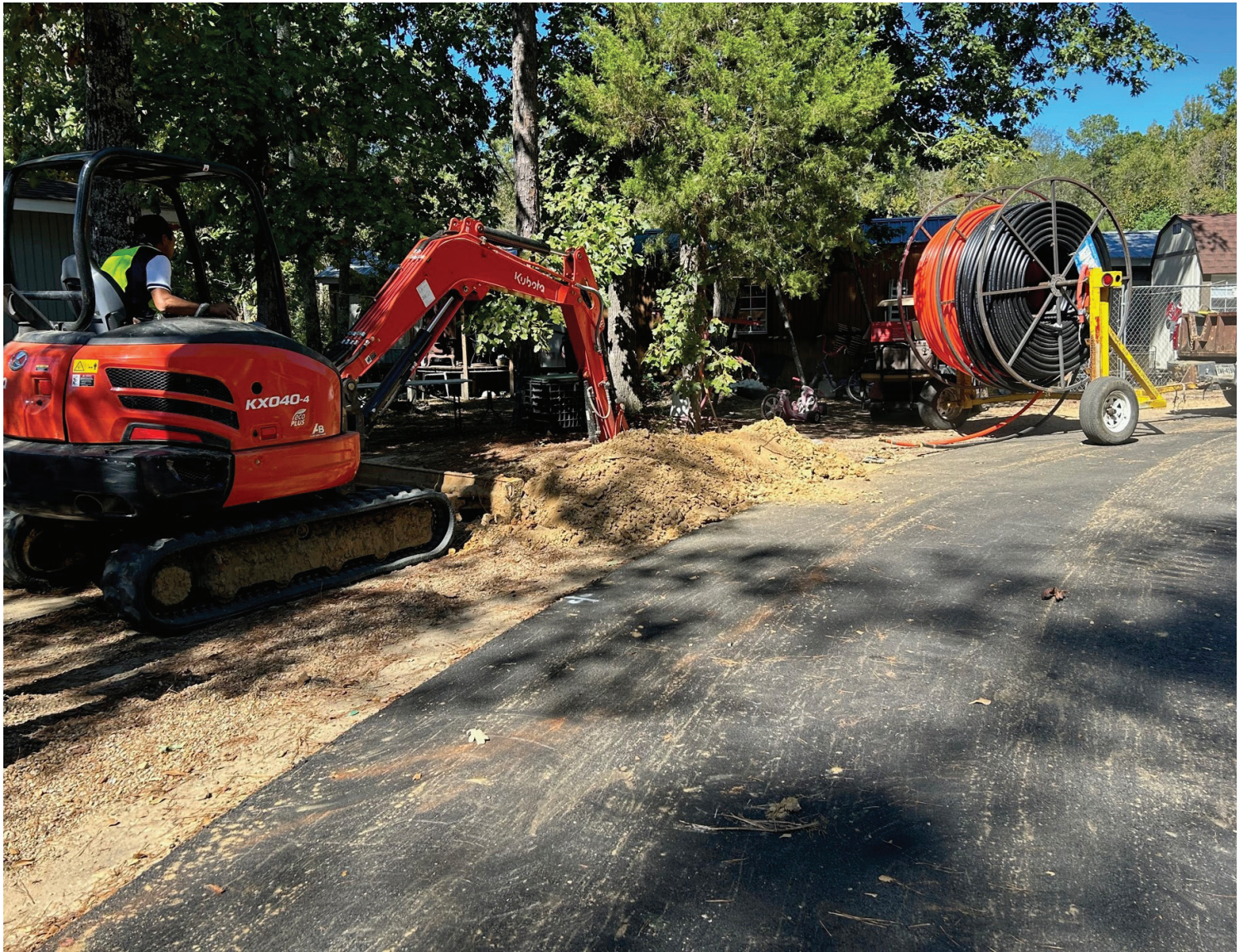
Franklin Telephone workers preparing to install buried fiber.
