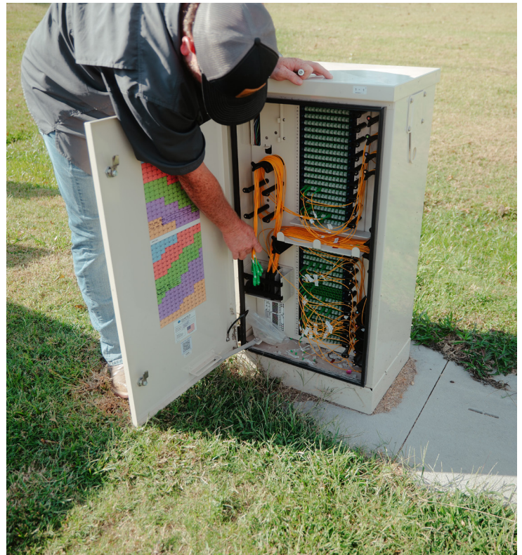
A representative of CSpire shows a fiber distribution hub installed as part of the Mayersville BIP project.
